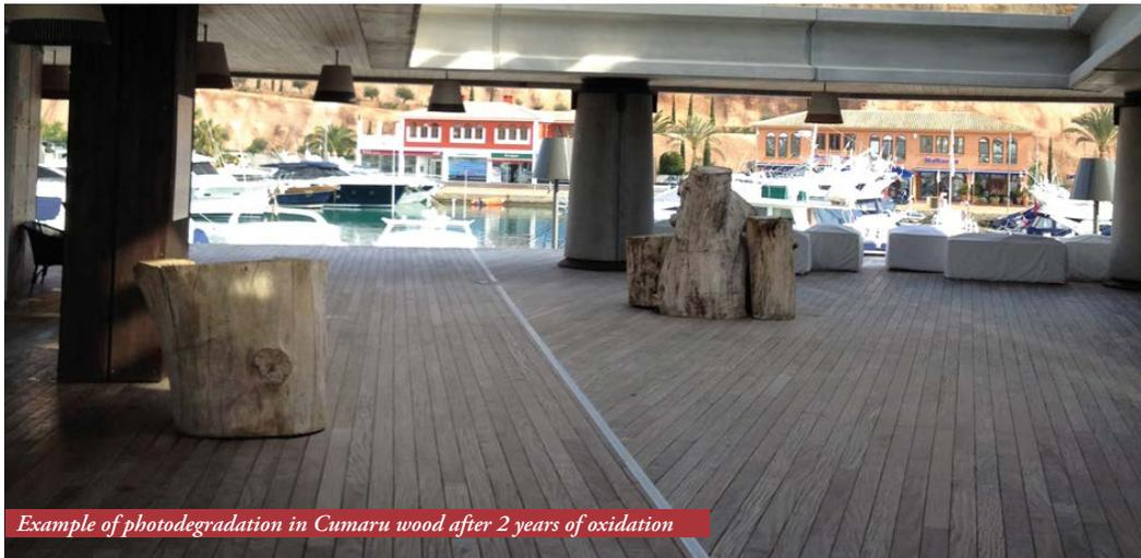
*Example of photodegradation in Cumaru wood after 2 years of oxidation*
