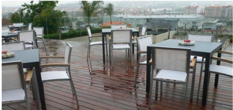
In any case, non-slip systems with continuous or mixed slotting must be used in order to reduce the slipperiness of the flooring when it is wet due to rainfall or splashing from pools, as recommended in Spanish standard UNE 56823:2008.
