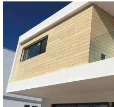
* You can see in page four an example of cumaru with two years of natural aging without maintenance, due to a correct installation.
